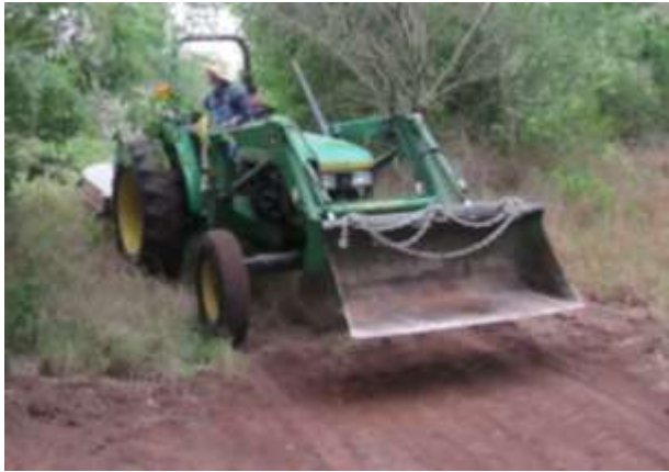
Apiary site is cleared and a gravel base is put in place to support the hives.
